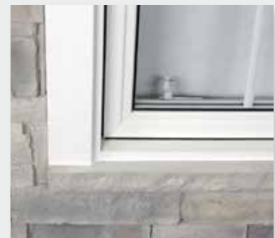
Finish with window sill, trim and jamb
